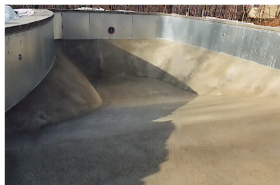
A typical vermiculite pool bottom just before the liner is installed.
